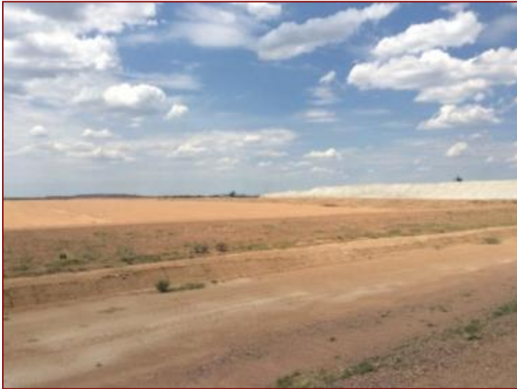
Figure 42- Image of the land dedicated to the facility and ash heap from Medupi power station. Taken from the south facing north-east
