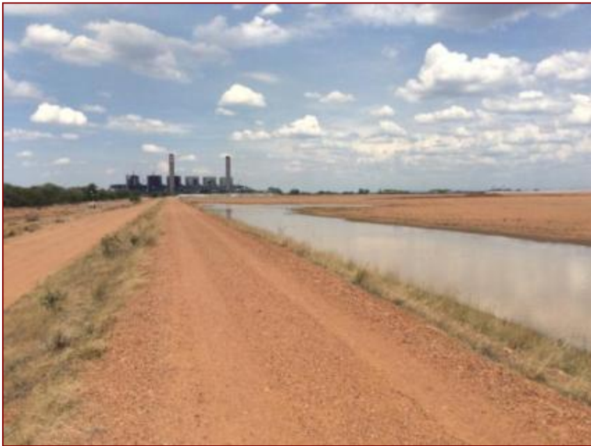
Figure 37- Northern end of the AFD
