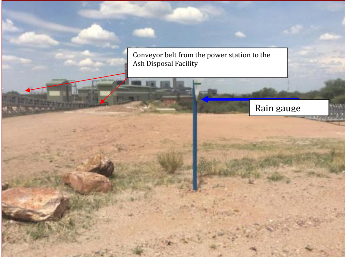
Figure 40- Conveyor belt system associated with the AFD
