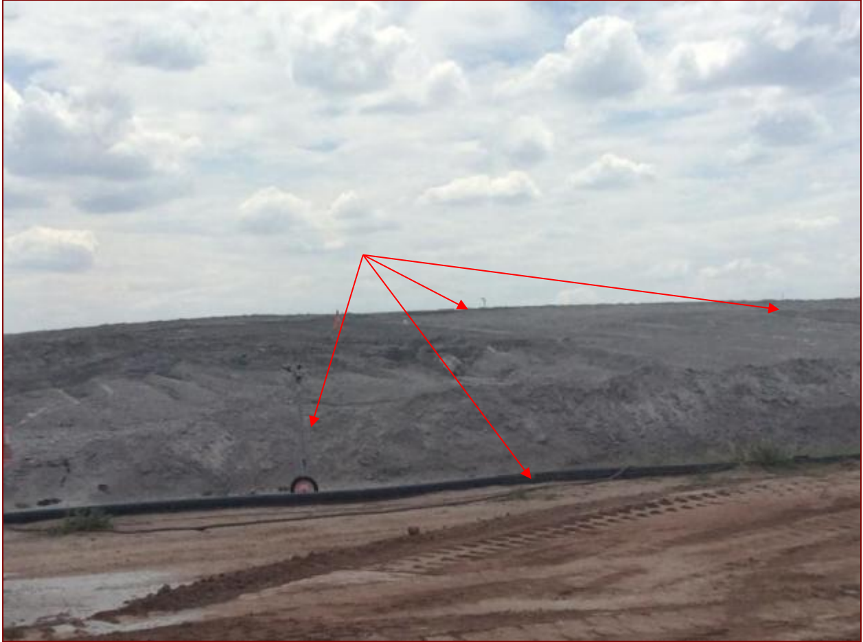
Figure 46- Sprinkler system developed to suppress dust
