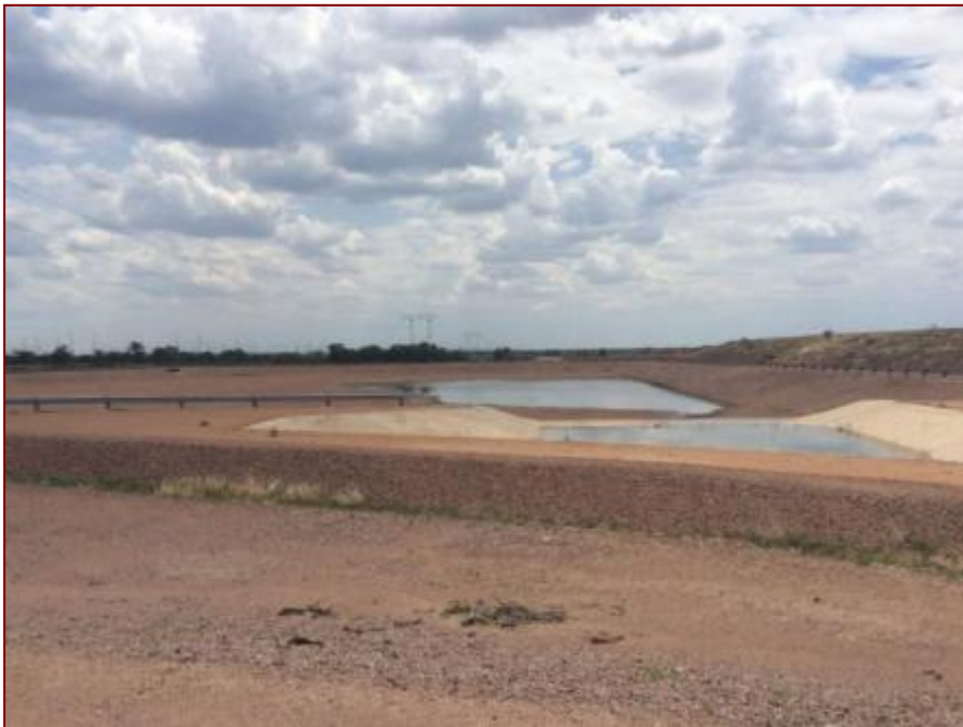
Figure 43- Two dams associated with the facility located south-west of the current ash heap
