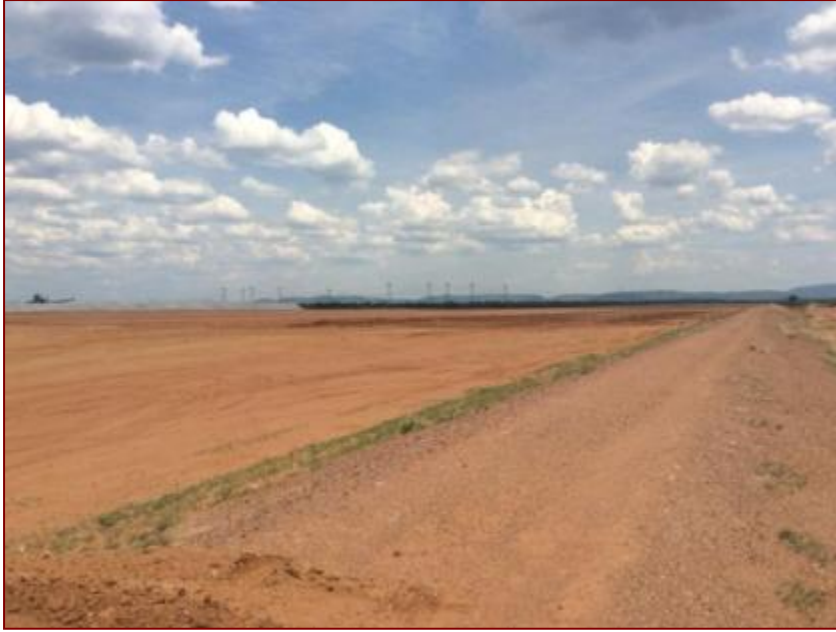
Figure 34- Available land that has been cleared for the growth of the Ash Disposal Facility (ADF). Image taken from the west facing east
