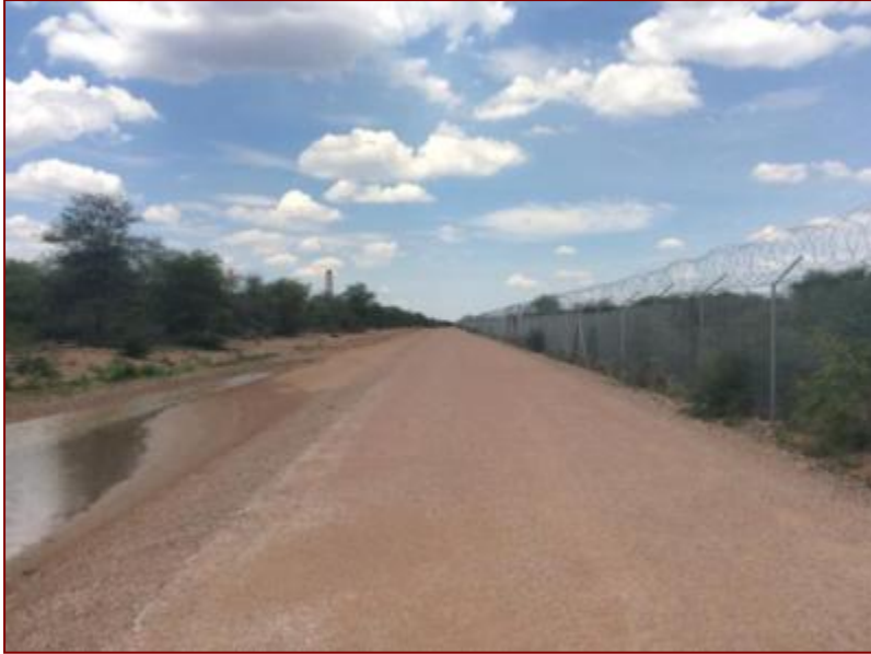
Figure 44- Fence line demarcating the facility with the southern property and the railway line
