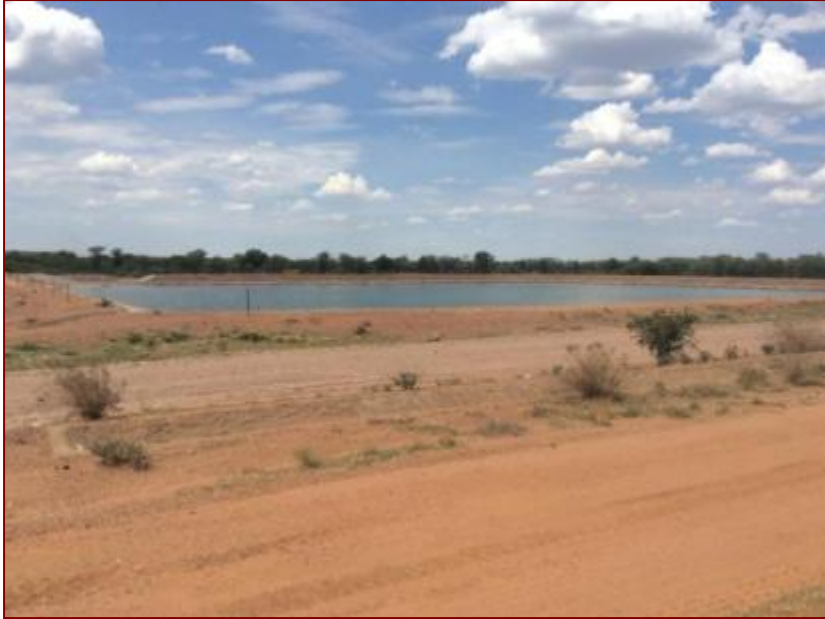
Figure 38- Northern dam associated with the AFD
