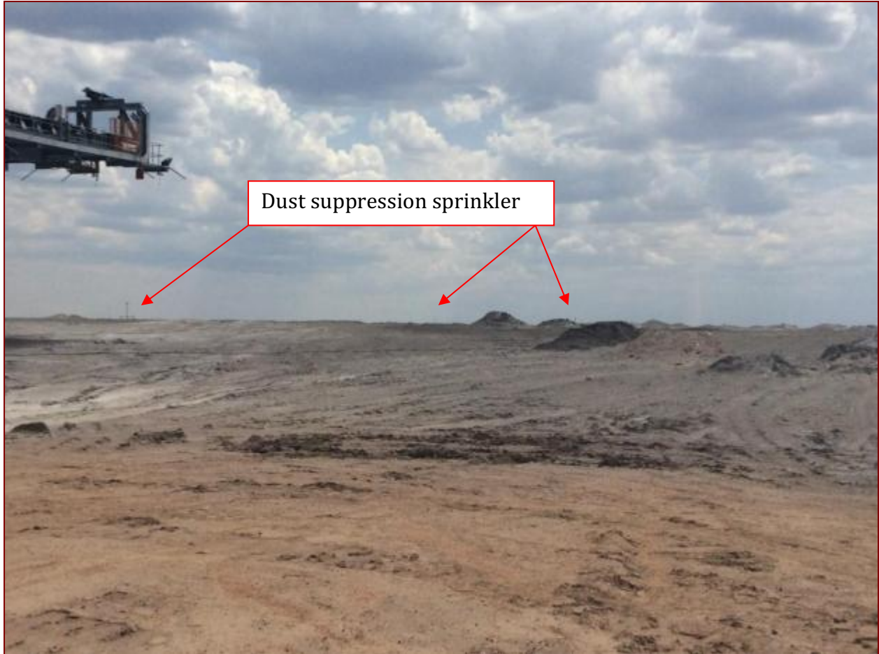
Figure 39- Current ash heap at the facility
